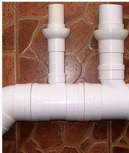
Water Heating Pipe Repair
