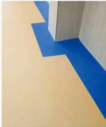
PVC Plastic Floor Construction
